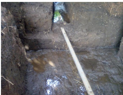
Catchment excavation at Njimoh
