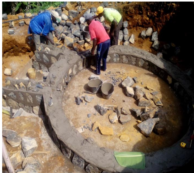
Casting of storage tank at Bamngam
