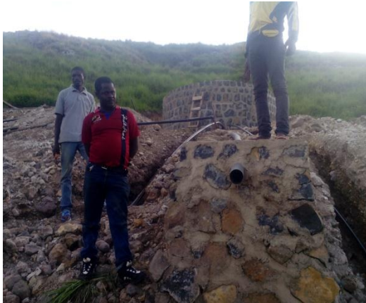
Kungi storage tank near completion
