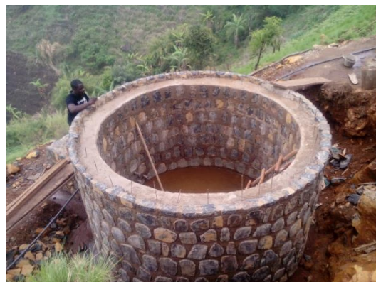
Moh storage tank under construction
